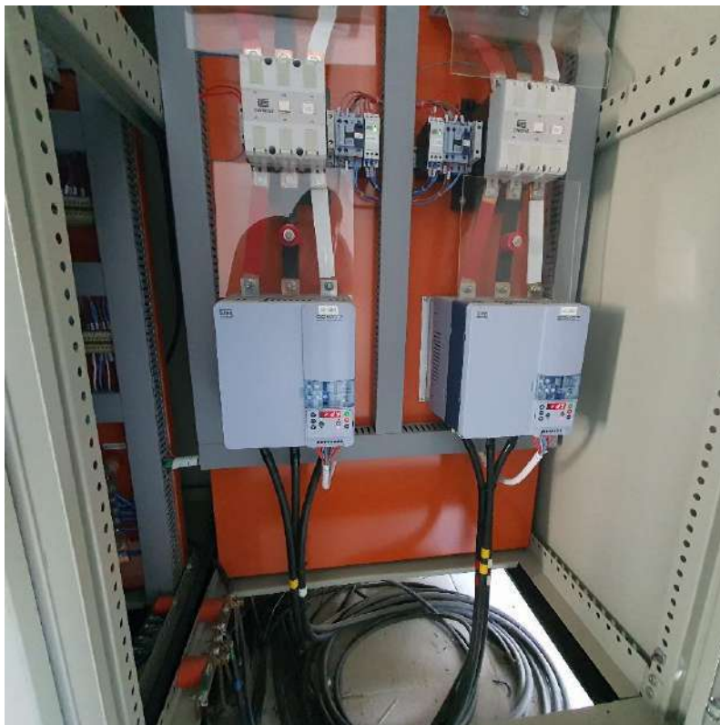
FIGURA 92 – SOFT STARTER EEEB BAGÉ
